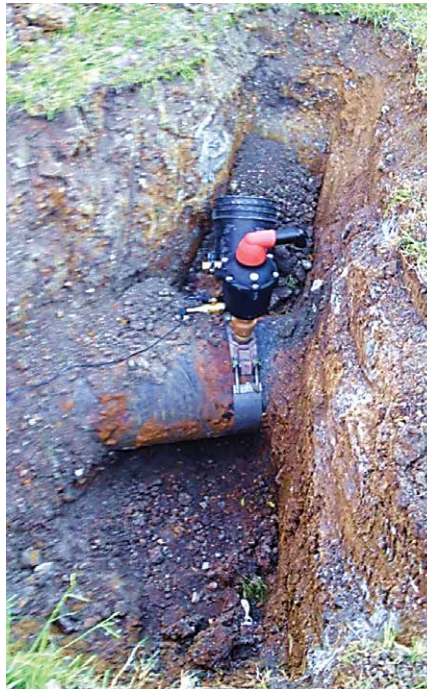
The 6-inch sewage air/vacuum replacement valve was put into service. Through transient monitoring data and computer surge analysis, it was determined that the valve was over sized, reacted too slow to the negative pressure wave, and discharged wastewater into the environment.
