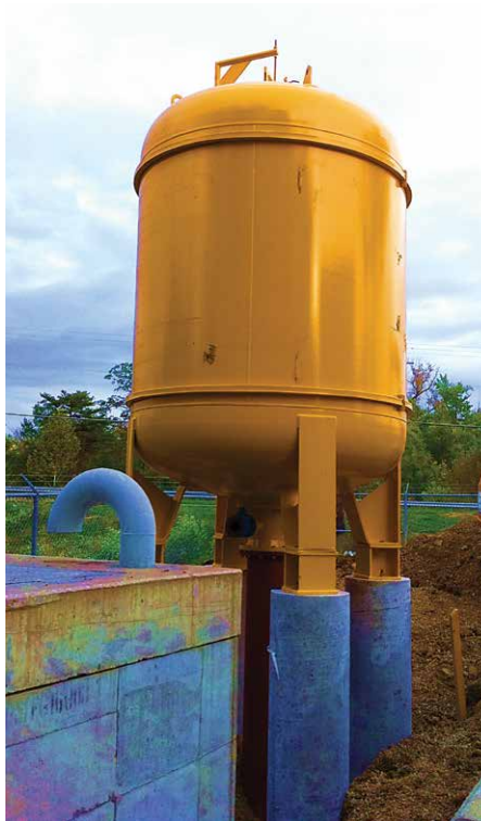
1,600 gallon Blacoh Bladder Type Sewage Surge Vessel designed to give energy to the change in velocity caused by the pump trip.
